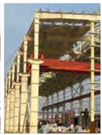
Pre-Engineered Building (PEB) is a metal enclosure building that includes a structural frame and standard roof and wall support which is factory made and is erected at the site. It is a new manufacturing concept replacing traditional manufacturing and providing custom-made solutions for both commercial and Industrial operations. PEBs are protected from sound and heat resistance. PEB weigh lighter and can effectively resist earthquake and wind pressure.
